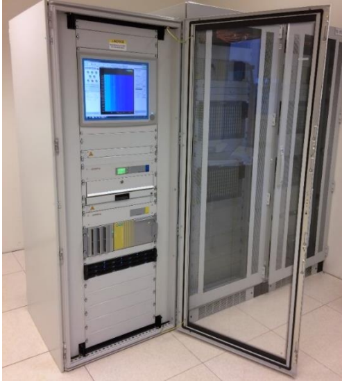
Fully integrated rack solution with DTS, DAS and SmartVision™ in the control room
